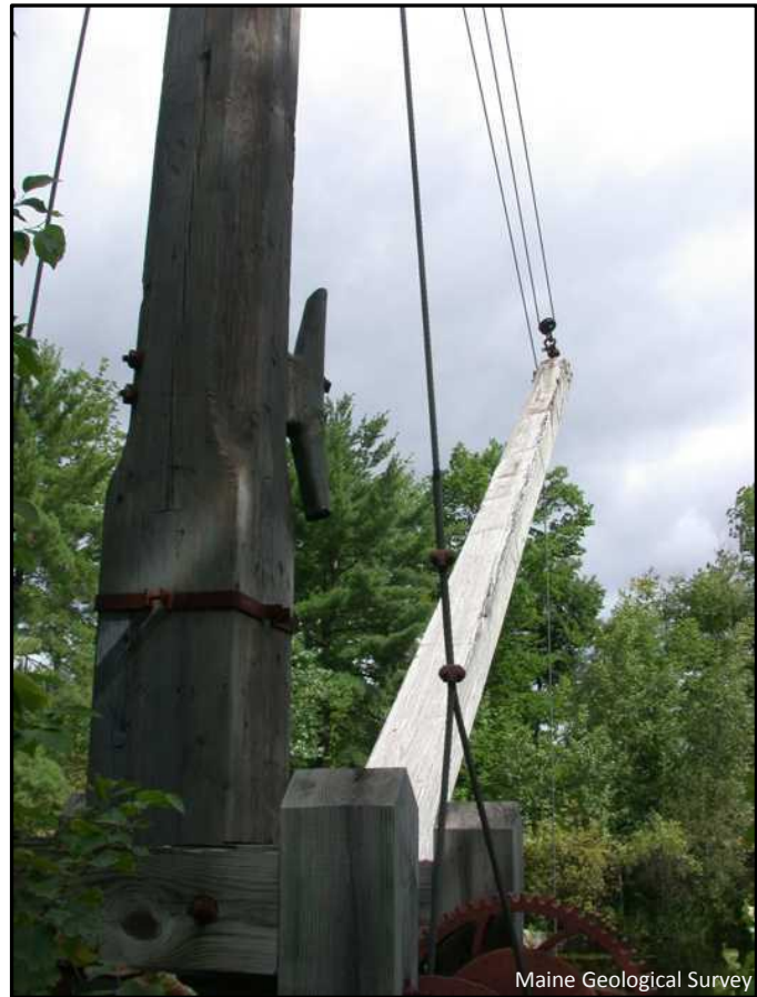
Figure 6. Derrick, Edison Drive, Augusta, Maine.
