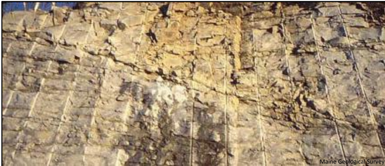
Figure 3. Large wall of granite blasted out during the construction of the adjacent national home improvement outlet (Area 2). The vertical stripes on the outcrop are from drilling to set dynamite charges. The nearly horizontal fractures are natural and carry the groundwater in this area, as shown by the icicle developed along one.
