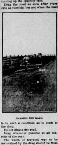
maintained by the drag should be from eighteen to twenty feet. First drag a little more than the width of a single wheel track, then gradually increase until desired width is obtained.
