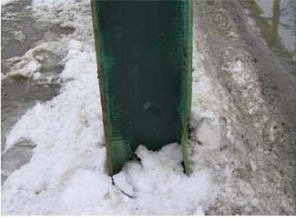
Damaged flange
