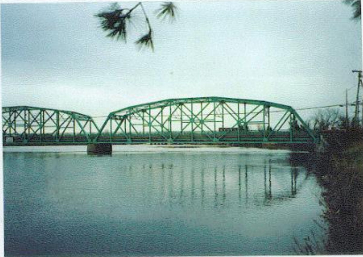
⑫ Bridge view from upstream
