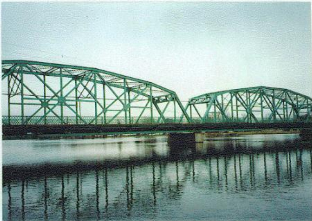
⑩ Bridge view from downstream
