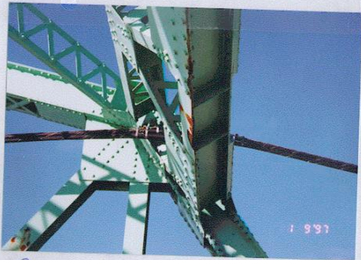
ABUTMENT 2 PORTAL COLLISION DAMAGE
