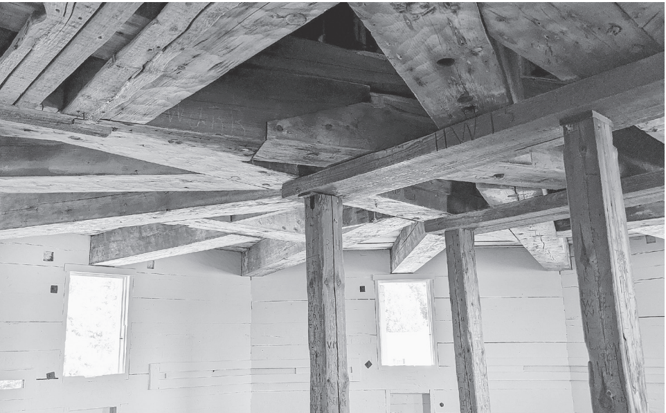
Fort Edgecomb — The amazing timberwork on the ceiling of Fort Edgecomb on Davis Island in Edgecomb. The intricate beams are the result of the octagonal shape of the blockhouse structure. PHOTO BY DAN KIRCHOFF
