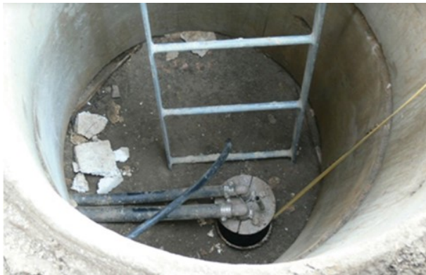
Figure 3. Well in well pit. Photo courtesy of Alberta Environment and Parks.
