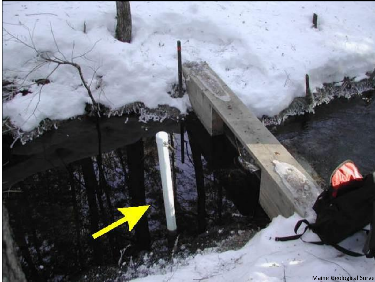
Figure 6. View looking downstream at 90 degree v-notch weir. Note location of pipe stilling well used for determination of upstream stage for flow correlation. Stream flow is calculated using water level measurements taken in the stilling well.
