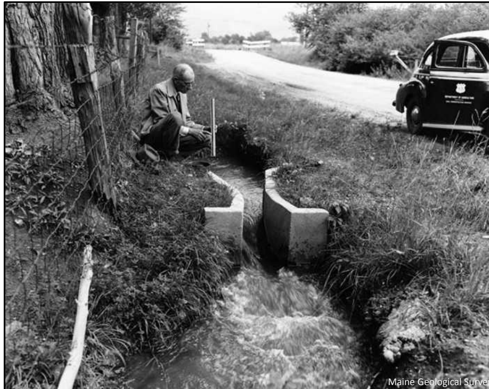
Figure 4. Dr. Ralph Leroy Parshall and the Parshall flume, 1946.
