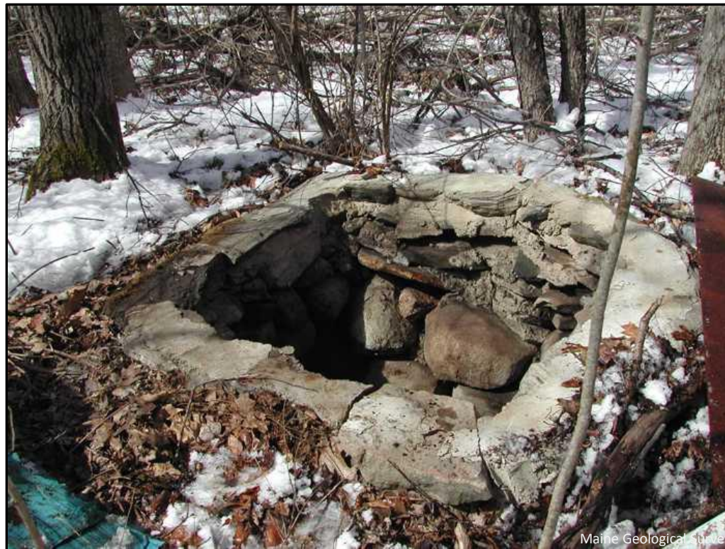
Figure 2. A hand-dug well lined with rocks in Richmond, Maine. This well has a total depth of 20 feet and is terminated on the bedrock surface. In the late summer, the water level is typically around 14 feet below land surface with a water column of 6 feet.
