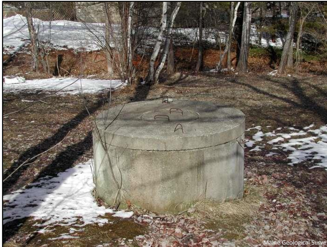
Figure 3. A backhoe-dug well with concrete tiles in Farmingdale, Maine. This well has a total depth of 12 feet. There are numerous springs in the area which contribute to recharge of the well. It does not go dry in the late summer.
