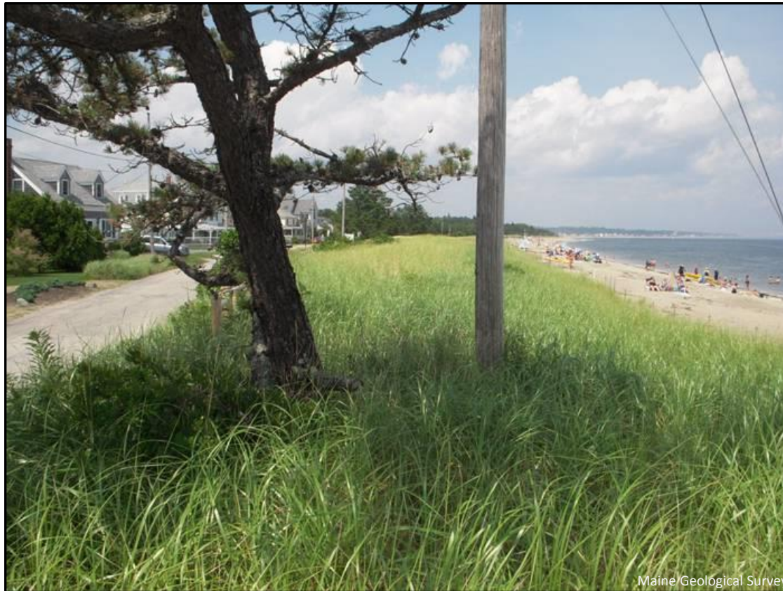
Figure 7. View north of secondary dune ridge constructed just north of the geotube project.
