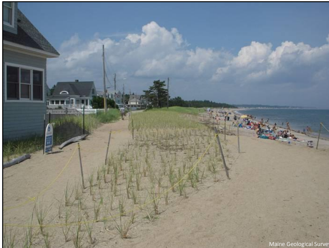
Figure 5. View north of geotube and dune grass plantings. The Ferry Beach Park Association's artificial dune construction begins at the tree and extends northwards (Figure 7).
