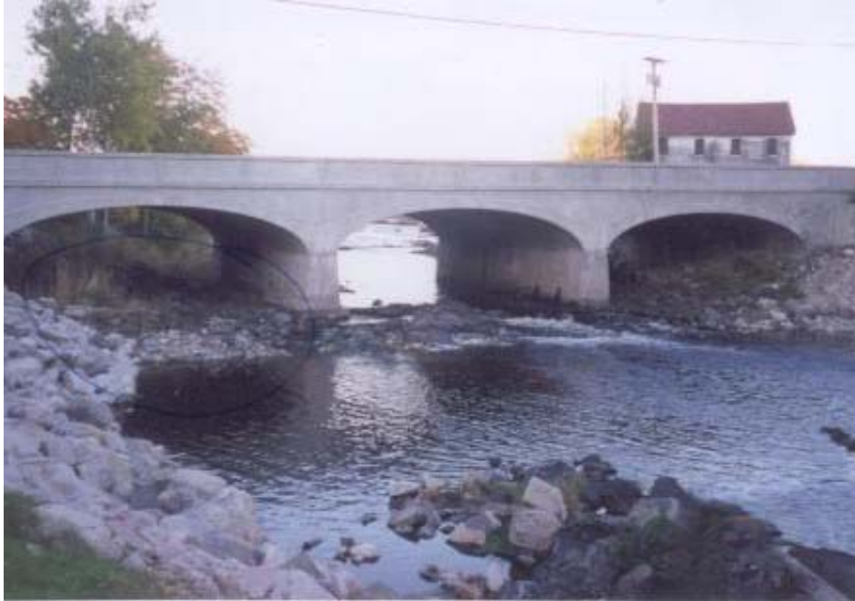
Pope Memorial Bridge, East Machias
