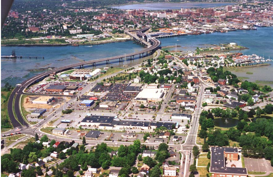
Casco Bay Bridge, Portland-South Portland
