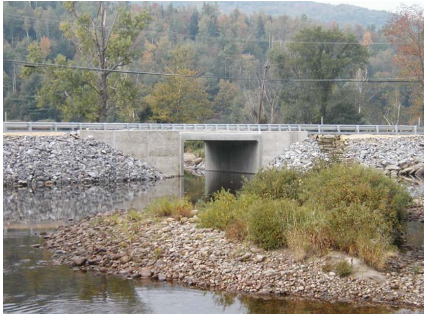
Scotty Richardson Bridge, Rumford
