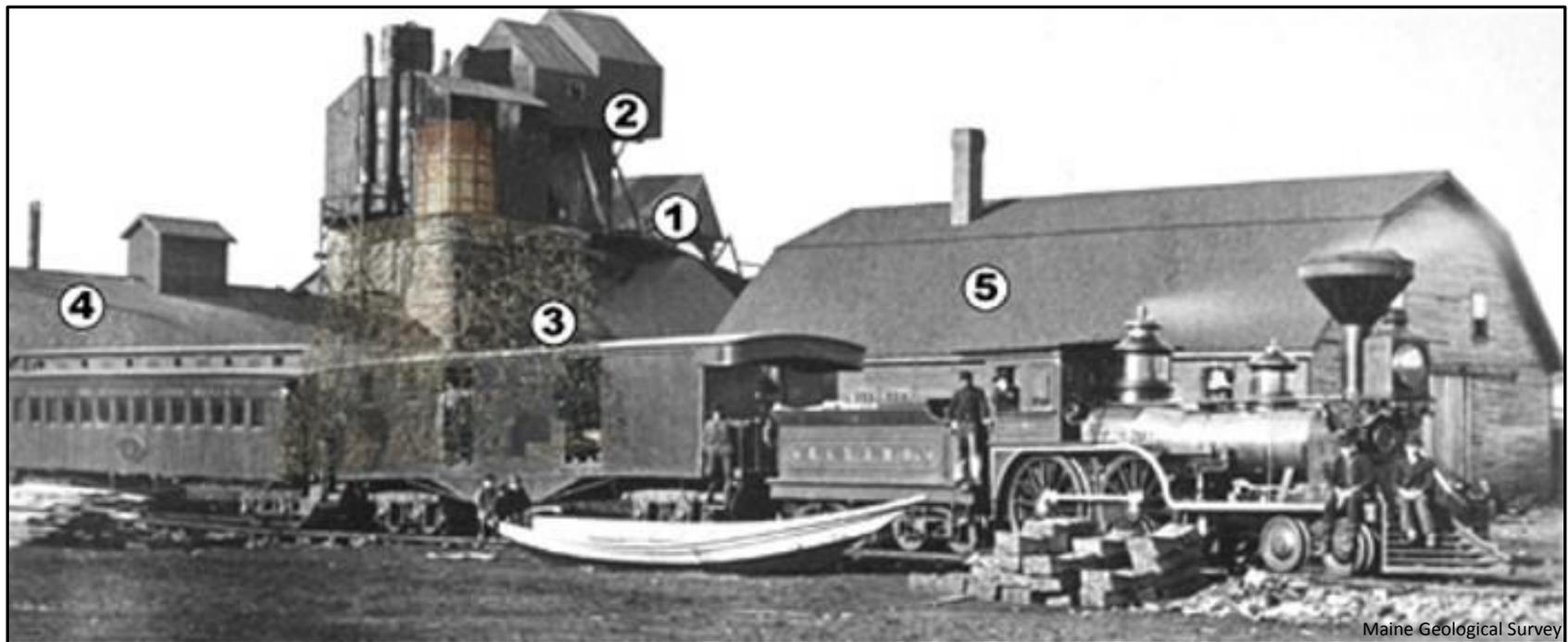
**Figure 5.** Building complex at Katahdin Iron Works showing ore kiln (1), top houses (2), furnace (3), casting shed (4) and storage barn (5) ([from Katahdin Iron Works website](#)).
