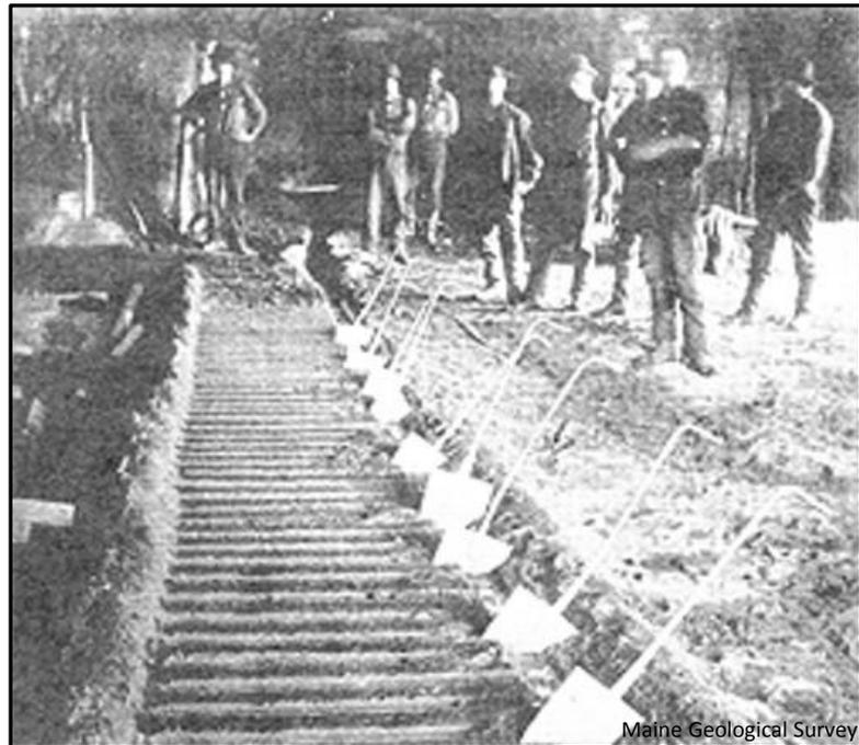
**Figure 7.** Casting house with pig-iron molds ([from Katahdin Iron Works website](#)).
