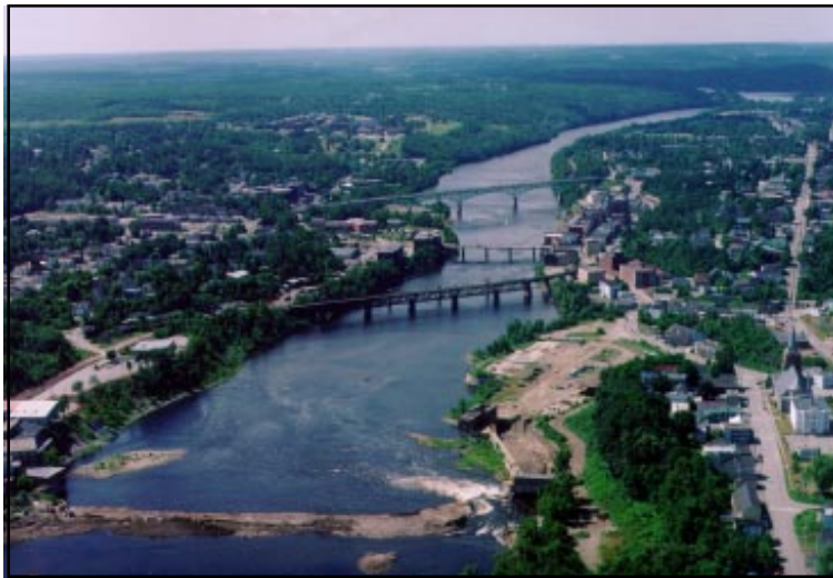
Edwards Dam Removal (looking south) Source: MDOT Photo Lab
