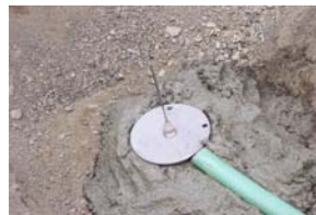
Soil Strain Gage Base Installed in Wet Concrete
