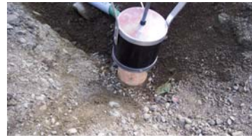
Removing the steel Plug for Pressure Cell Installation Method 2
