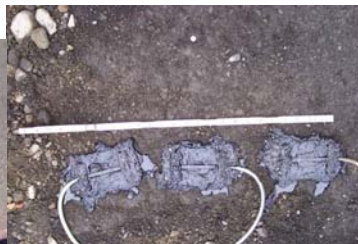
Asphalt Strain Gages Ready for Paving
