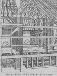
are 2 by 8, the joist beams 2 by 10, and the braces are of the lighter timbers This barn is 40 by 80 feet, with 24 foot posts. There is a basement 8 feet high throughout the entire building, with a 12 foot driveway through the center the short way.
