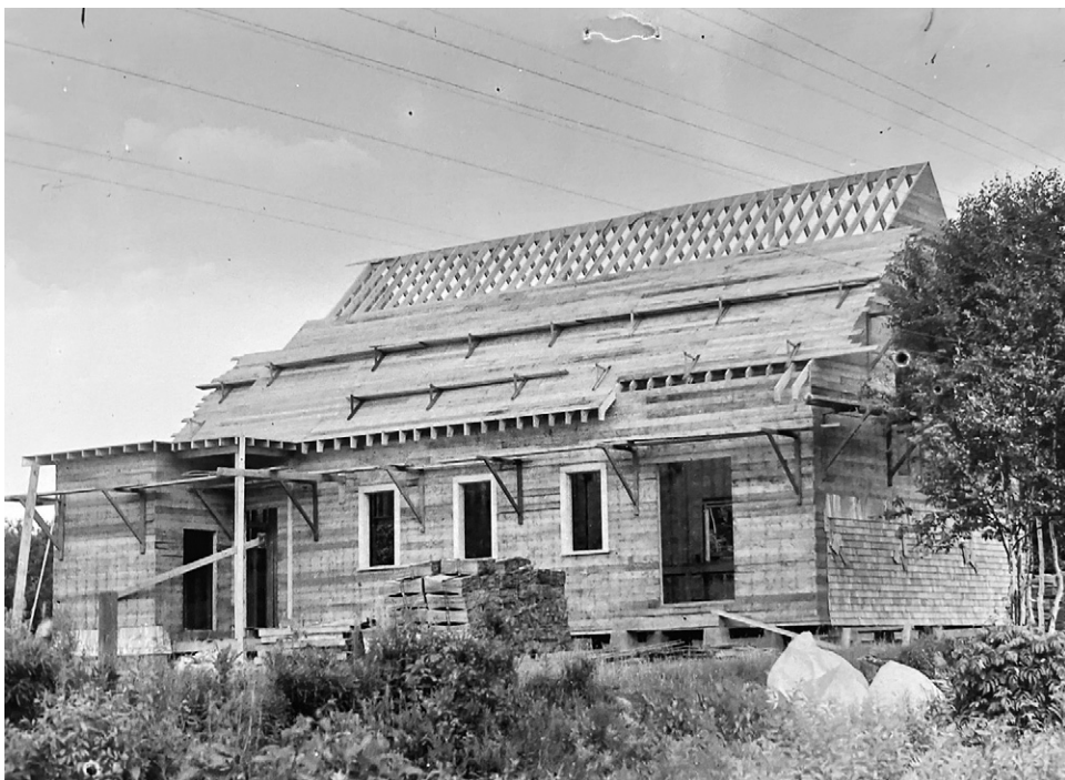
Seen here is the framed building being sheathed with rough sawn boards and covered with cedar shingles. Note the stacked bundles of shingles in the work area. Keep in mind that carpenters in those days used hand saws and good old hammers.
