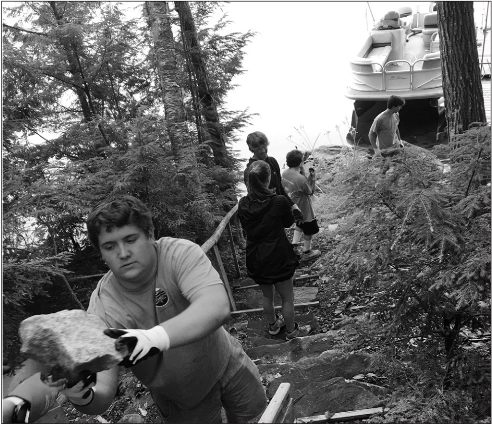
YCC moving rock toward shoreline to install an erosion control measure to keep phosphorus out of the lake.
