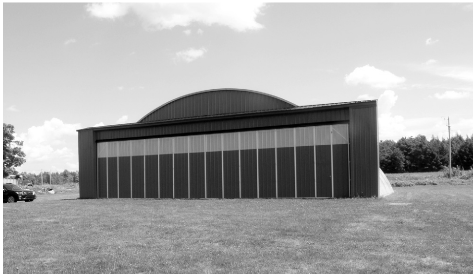
Large prefab steel hangar with vertical accordion folding doors .
