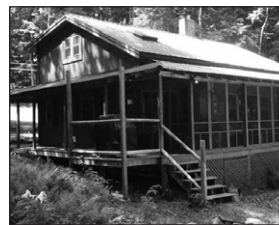
PARKER POND, CHESTERVILLE: 3 Season, 4BR/1.5BA, screened porch, oversized farmer's porch, outside shower, completely renovated in 2001. #1209443 $375,000
