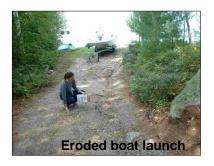
Due to the nature of their design and purpose, boat launches also tend to direct runoff into lakes. Typical problems observed on boat launches in watershed surveys include surface erosion, poor surface material and shoreline erosion. Even lakes with public boat launches commonly have several, if not dozens, of private launches.
