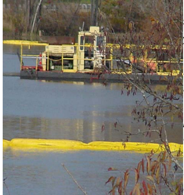
Figure 43. The dredging barge used to remove sediment and pump it to the processing location.
