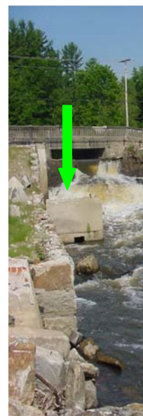
Figure 40. Hydraulic conditions during high flows that Sabattus River staff located at the upstream passage at the Juliet Dam, indicated by the green arrows.
