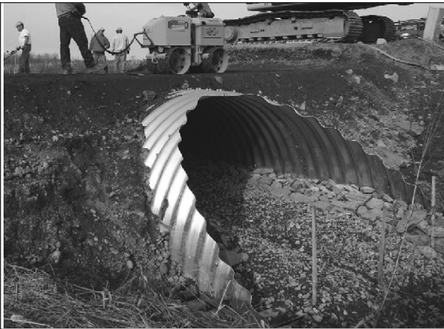
This culvert seems large enough to allow a stream channel to form in the bottom.
