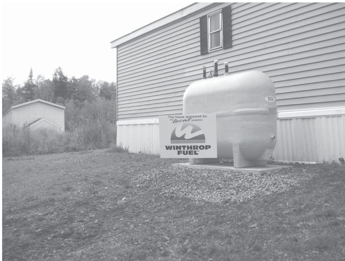
Newly installed double wall home heating oil tank
