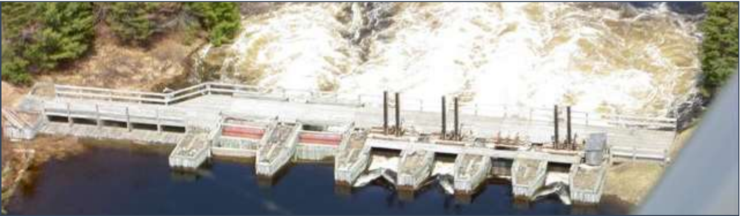
Aerial View of Telos Dam by AWW Chair, Rick Denico
