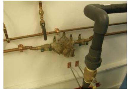
*A testable backflow prevention device on a treatment feed line*
