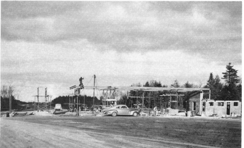
Portland toll houses under construction – 1947.
