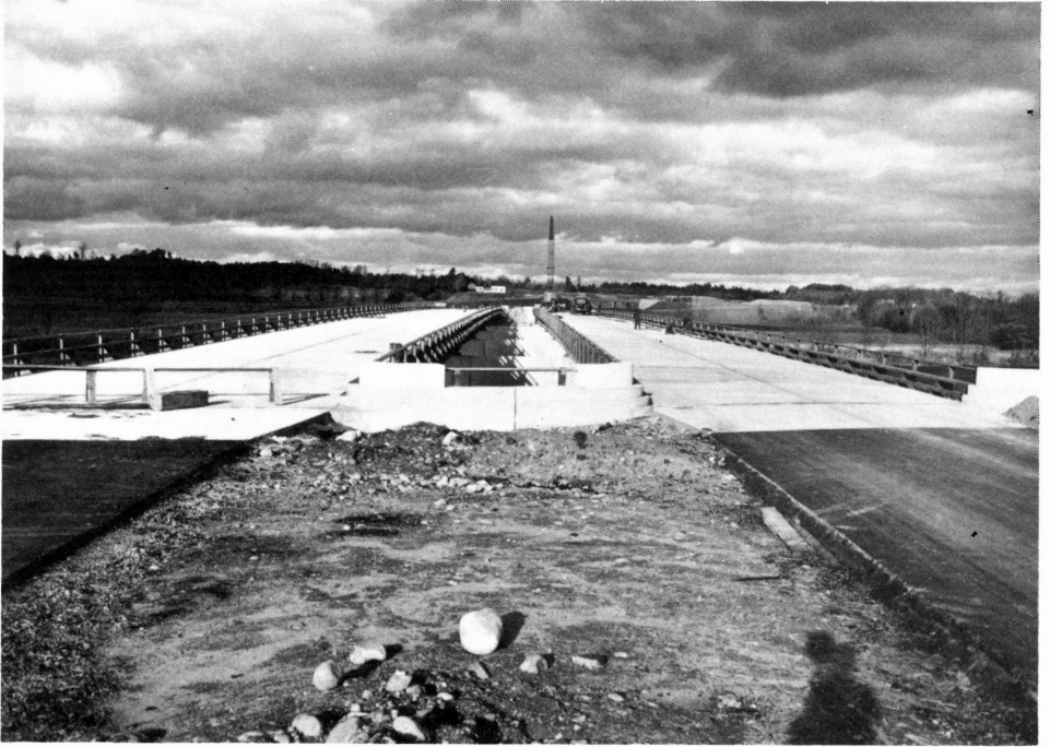
Decking over the Saco River Bridge, Nov. 1947.
