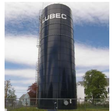
Security fence with locked gate around storage tank
