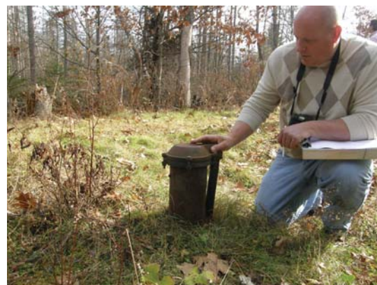
Field Inspector Greg DuMonthier inspects the well of a small water system during a sanitary survey
