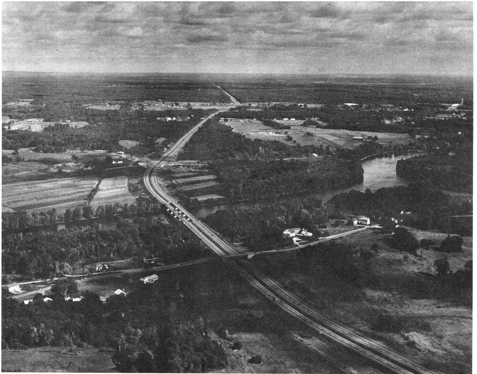
SECTION I - SACO RIVER BRIDGE
