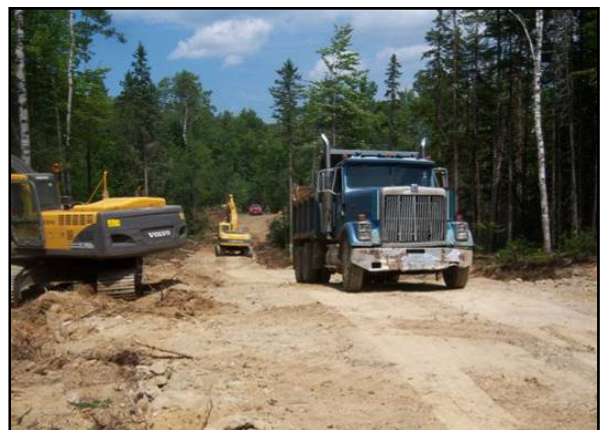
Management Road Construction at Nahmakanta
