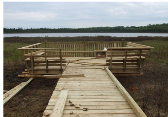
Salmon Brook Lake Bog observation platform during construction
