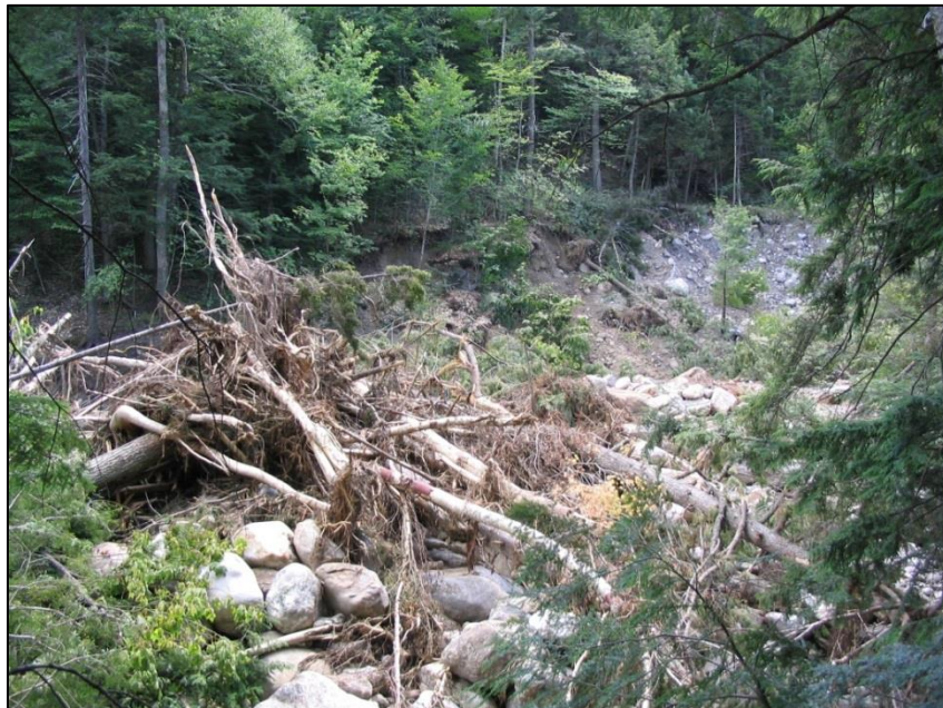
Figure 5.2. Debris swept down Chapman Brook in Bethel by the deluge of 2007. A town reservoir was filled with boulder gravel by this event.
