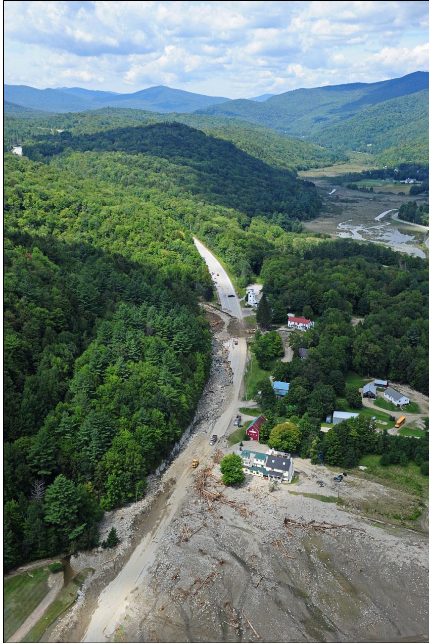
Figure 5.4. Property overwhelmed by flood deposits from tropical storm Irene in 2011, Routes 4/100 south of Killington, Vermont. Photo by Lars Gange & Mansfield Heliflight.
