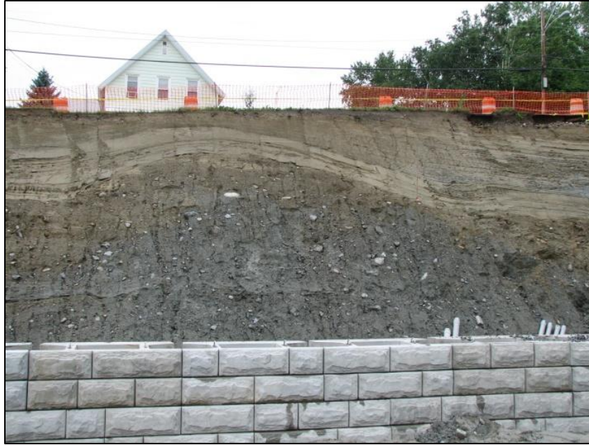
Figure 3.18. Clay-silt beds (Presumpscot Formation) draped over stony till (probable moraine), at same Augusta site as Figure 3.17.
