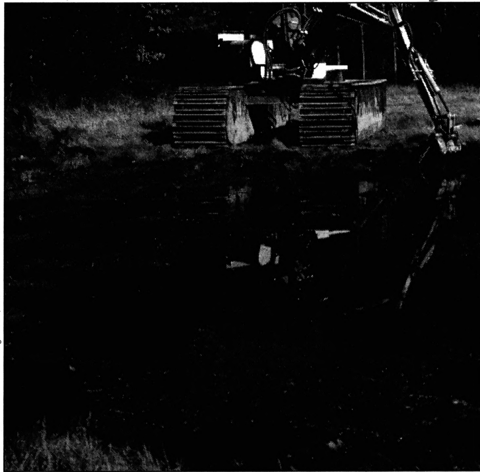
As part of the Great Bay salt marsh restoration project, an excavator creates a pond hole to restore open water habitat to the marsh surface.
