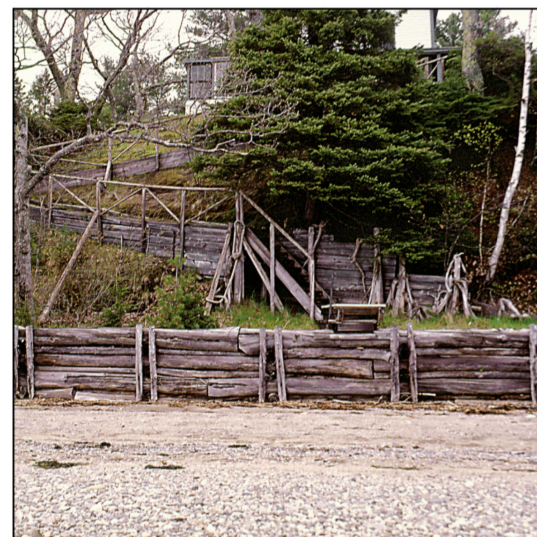
Stable bluff with a vegetated bluff face and an armored shoreline. The bluff face is fully vegetated and supports a mature stand of trees with vertical trunks. The presence of a wooden bulkhead suggests that erosion has occurred in the past.
