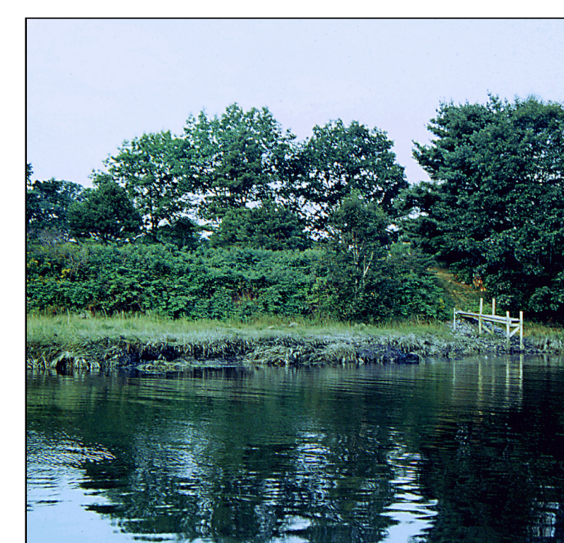
Stable bluff with a vegetated bluff face and a salt marsh shoreline. A low bluff face is covered by shrubs landward of a salt marsh terrace. In this location the mature marsh protects the base of the bluff from rapid erosion and slows bluff recession or retreat.
