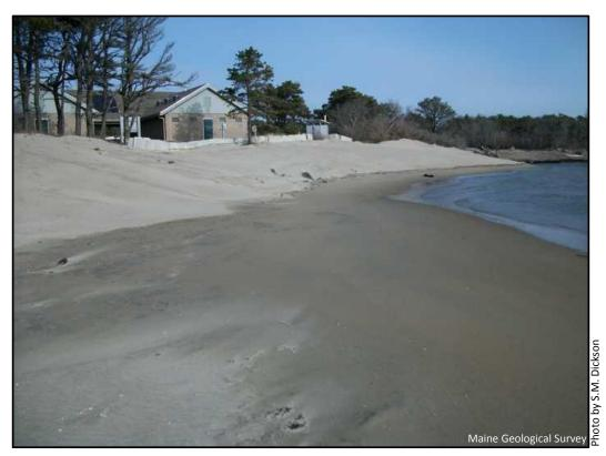
**Figure 10.** A view of the new beach face seaward of the bath house four days after it was created by beach scraping. Wind and wave action is gradually removing the tracks from the bulldozer. The tree wattles and vertical dune scarp are covered with sand. The recent high tide line is delineated at the upper reaches of the wet beach.
