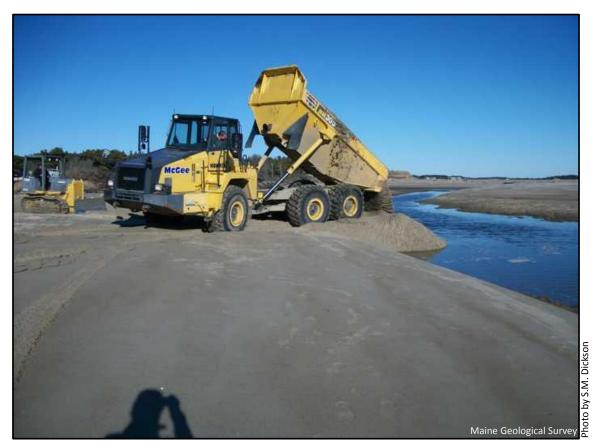
Figure 9. Sand from the spit was loaded into dump trucks and used to fill the tidal channel.
