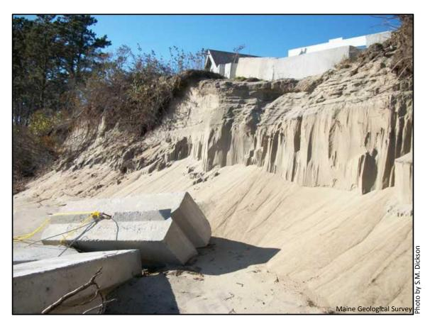
**Figure 4.** Ongoing erosion of the bank and sand immediately seaward of the bath house resulted in cement blocks being undercut and falling into the tidal channel.
