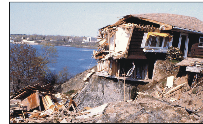
Figure 1. A clay bluff on the north shore of Rockland Harbor failed in 1996. This landslide formed a new scarp about 200 feet landward of the original top of the bluff in just a few hours. Two homes were destroyed as a result of this catastrophic slide (see Berry and others, 1996).
