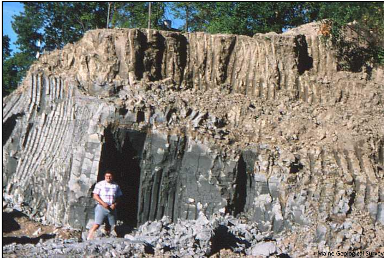
Figure 5. Construction site in Gardiner showing exposure of oxidized and non-oxidized clay.
