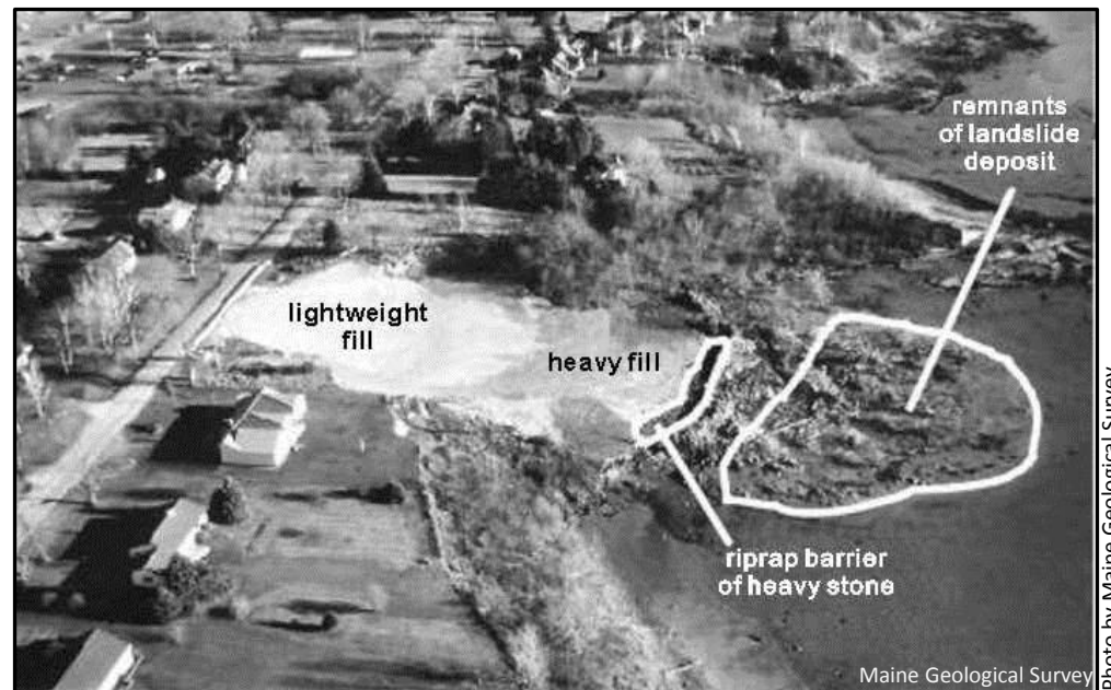
Figure 3. Photo of the Rockland landslide project showing locations of lightweight cement kiln dust, heavy rock fill, and the riprap barrier. The remnants of the slide on the tidal flat will be allowed to gradually erode.
