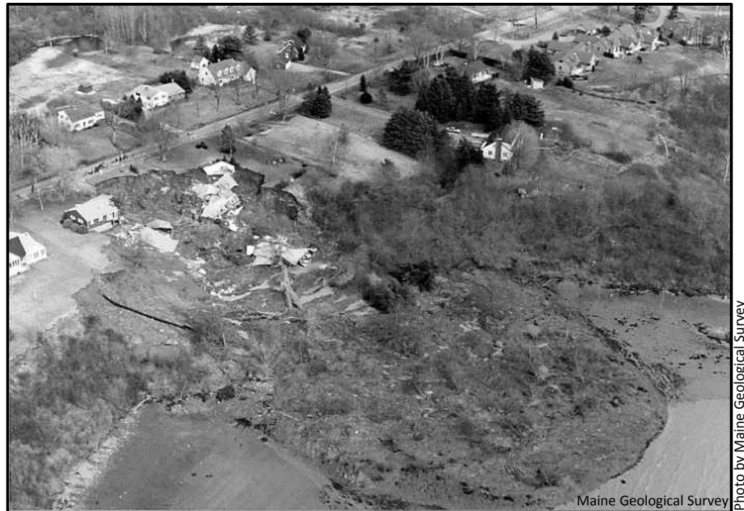
Figure 1. Air photo of the Rockland landslide, April 1996.
