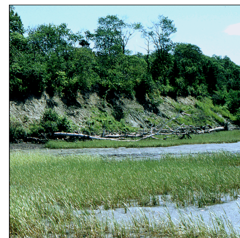
Highly unstable bluff with an unvegetated bluff face and a salt marsh shoreline. Sediments on the bluff face are exposed and fallen tree trunks lie at the base of the bluff. A salt marsh has recently formed on the tidal flat, partly on the top of an old landslide deposit.
