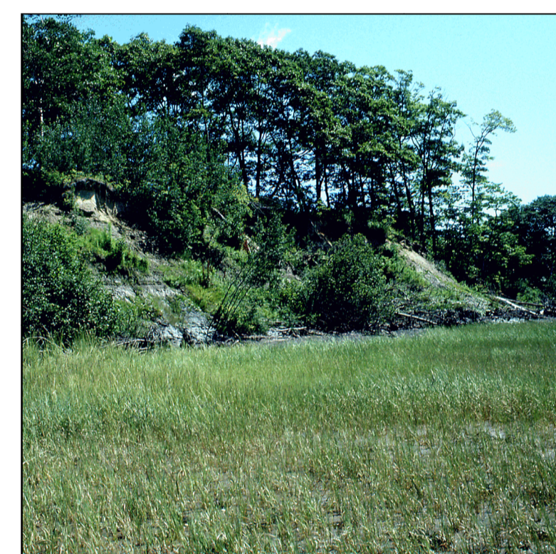
Unstable bluff with a partially vegetated bluff face and a salt marsh shoreline. This bluff, protected by a salt marsh, remains unstable. There are small bushes on the bluff as well as small non-vegetated areas that indicate continuing bluff retreat.
