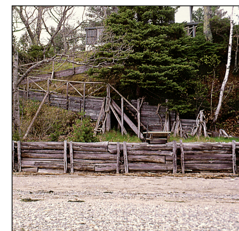
Stable bluff with a vegetated bluff face and an armored shoreline. The bluff face is fully vegetated and supports a mature stand of trees with vertical trunks. The presence of a wooden bulkhead suggests that erosion has occurred in the past.
