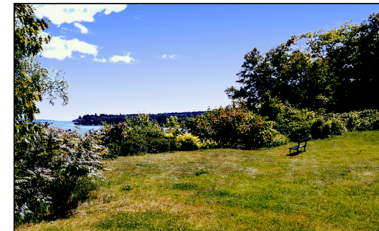
Figure 3. The shape of the top edge of a bluff can be an indicator of landslide risk. Clay bluffs often fail at points of weakness. Such a "slump" can expand into a larger landslide that cuts into the bluff and forms a curve around the original point of failure. Multiple slides and slumps will form an irregular or arcuate top edge to the bluff as shown in the photo above. Bluffs made of coarse materials or sand have a more even upper edge caused by a more constant rate of erosion along the bluff face.
