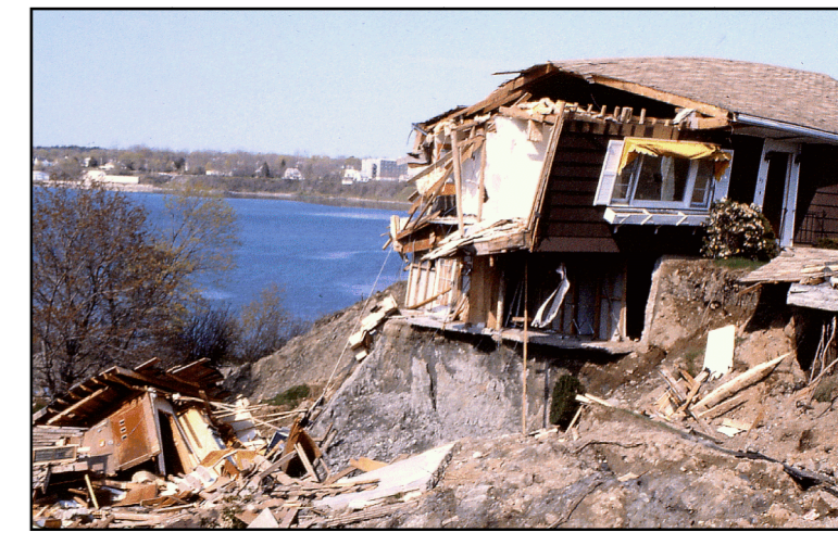
Figure 1. A clay bluff on the north shore of Rockland Harbor failed in 1996. This landslide formed a new scarp about 200 feet landward of the original top of the bluff in just a few hours. Two homes were destroyed as a result of this catastrophic slide (see Berry and others, 1996).
