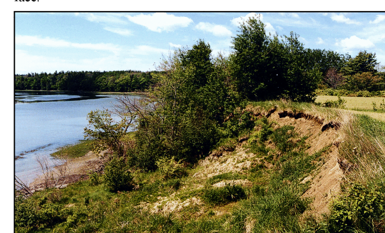
Figure 5. Terraces or a hummocky land surface on the slope of a bluff can indicate a former landslide. Terraces on the bluff face contribute to surface water flow and destabilize the bluff. In addition, a high water table can saturate and weaken muddy sediment and make the ground more prone to slope failure.
