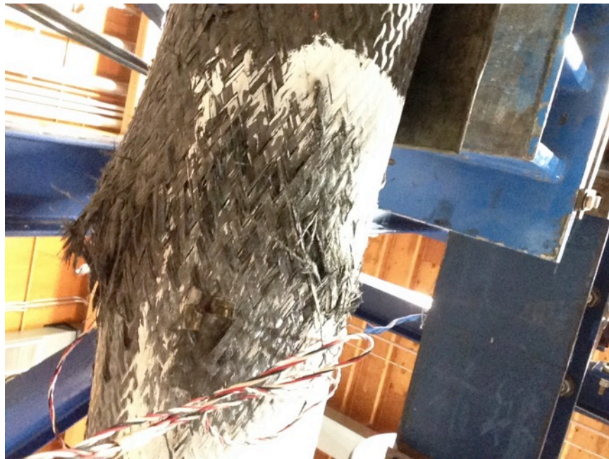
Figure 16 – Tensile Rupture of FRP near Midspan
