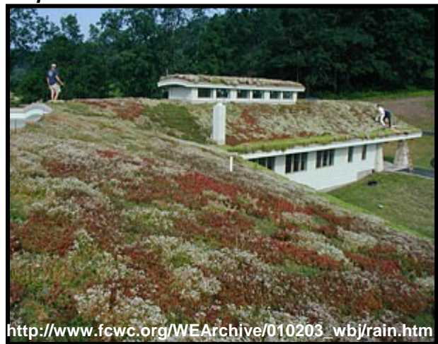
Figure 2: Green roof installed on a sloped roof
