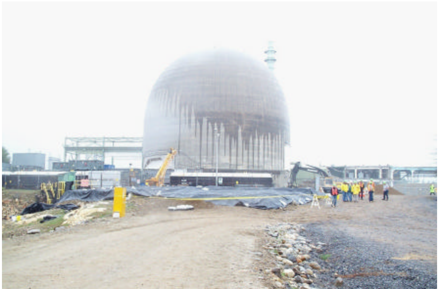
Deconstruction is well underway at Maine Yankee.
