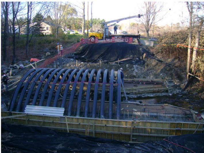
One such example is the Neal Bridge in Pittsfield which was constructed in the fall of 2008. The 27 ft. long arch structure was manufactured from hollow carbon fiber composite tubular arches spaced at approximately 2-feet on center, erected in place and filled with concrete. A corrugated fiber reinforced plastic (FRP) composite decking was installed on top. The head walls were constructed with a FRP sheet pile system.
