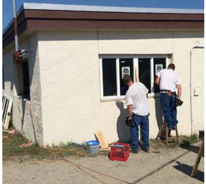
Downeast Correctional Facility work crew inmates replaced the windows in Dorm III this summer.
