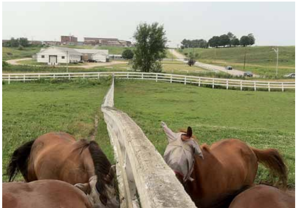
Maine State Society for the Protection of Animals fencing in need of repair.
