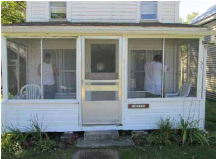
MDOC work crews tackle a chore list of more than 70 items.
