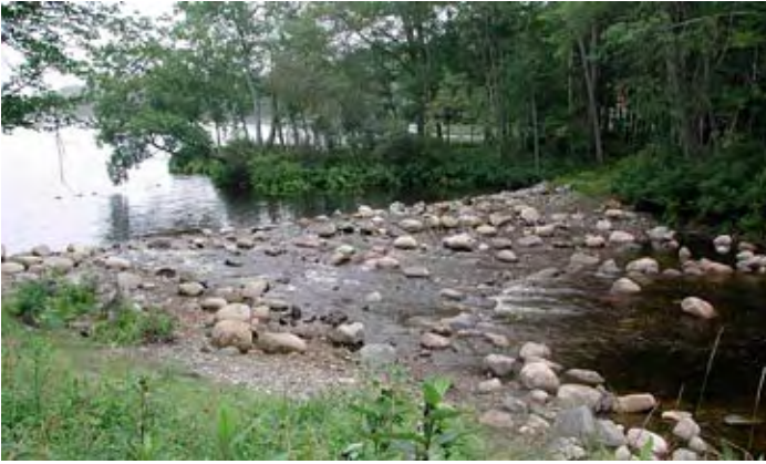
Rock ramp at the outlet of Sennebec Pond in Union, Maine, which replaced a dam but still maintains pond levels. Eric Hutchins
