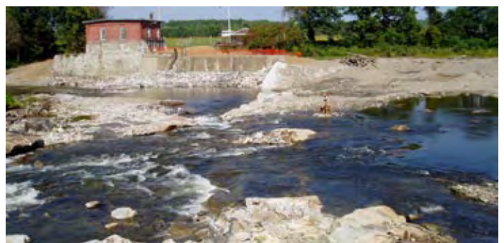
Removal of the Madison Electric Works Dam on the Sandy River in Norridgewock, Maine. The dam was removed in the summer of 2006, allowing diadromous fish access to the watershed of Maine's 12th largest river. Eric Hutchins
